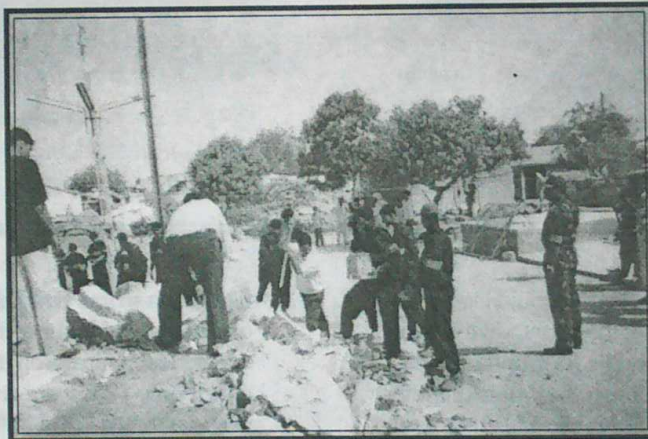
RIMC Cadets Removing Debris At Bhuj
